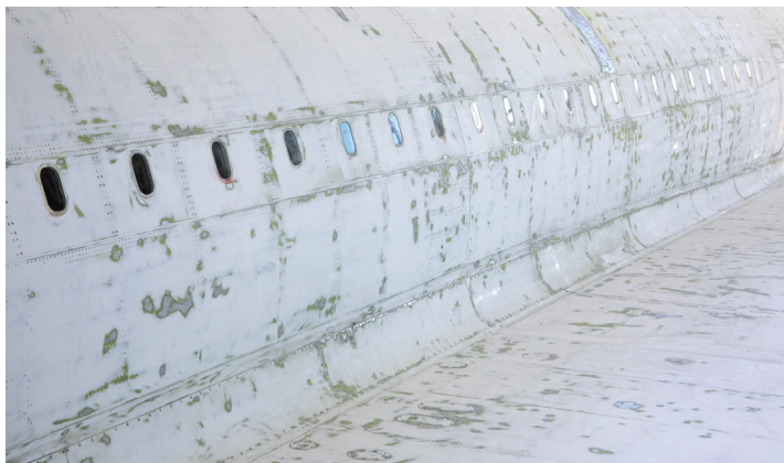
Preparatory work Above: The fuselage and wings, after many days of sanding and priming work. Photo: Ted Huetter/ The Museum of Flight
